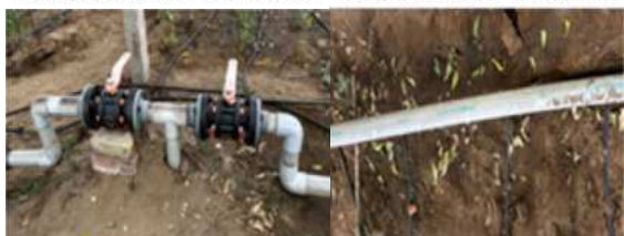
Sub-mains connected to valves sub-mains connected to laterals
