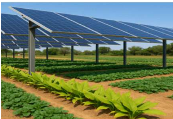
Figure 1: Pilot project in India showing elevated solar panels with crops like turmeric and spinach cultivated beneath
