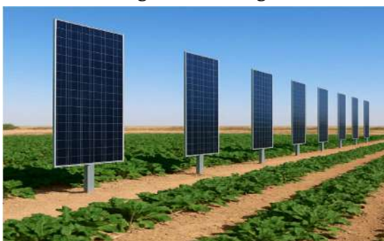
Figure 1: Example of vertical AgriVoltaic system used in arid regions (Tunisia). Panels are mounted vertically between crop rows to optimize space and solar capture.
